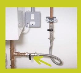
Tap to boiler **slowly** open to allow water into the heating system.
