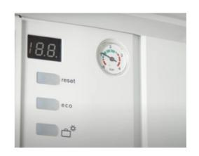
Do not overfill the pressure past 1.5 bar on the gauge as it could damage the boiler and system.
