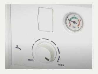
Keep a careful watch on the gauge. Once the pressure reaches just past 1 turn off both taps.
